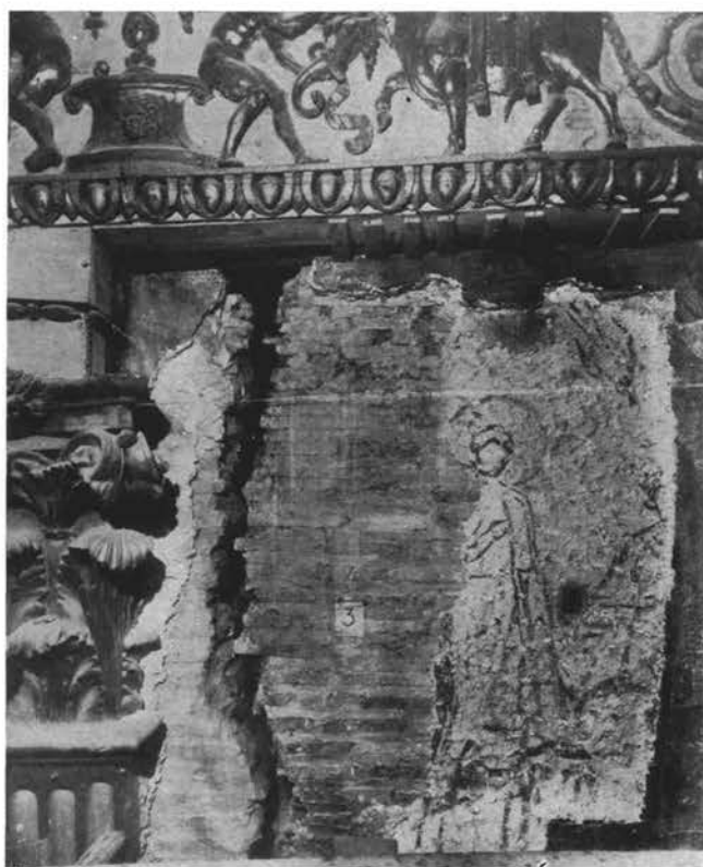
Fig. 47. S. Maria Maggiore, Triumphal arch, south spandrel, detail of brickwork and sinopia
